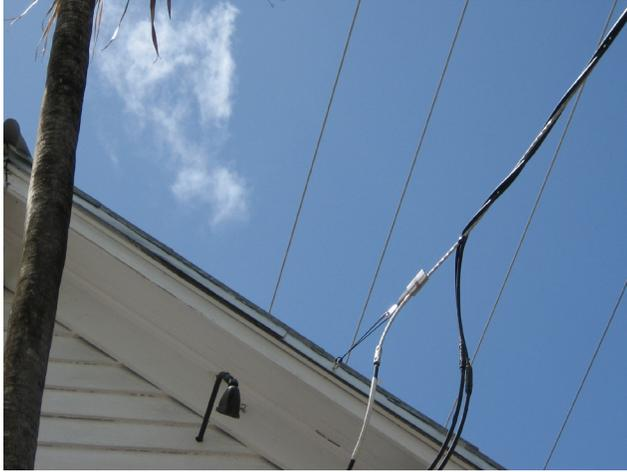
Wedge clamps are mechanical holding devices used for strain relief in service applications.
